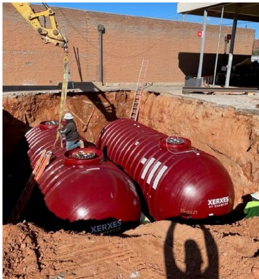
New, underground fuel tanks at Gashopper Stopper/Conoco
